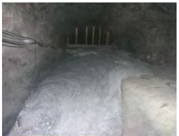
Typical underground hydraulic backfill
