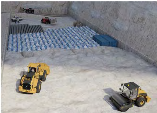
Open cut kaolin mine creates the voids (left). The voids are used for the safe and secure storage and permanent isolation of waste in sealed containers (right).
